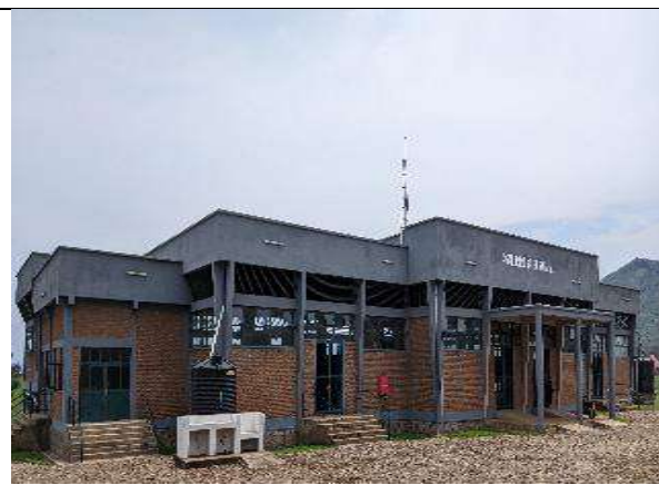
Bugarama handcraft workshop not yet used. Photo taken by OAG on 19 October 2023
